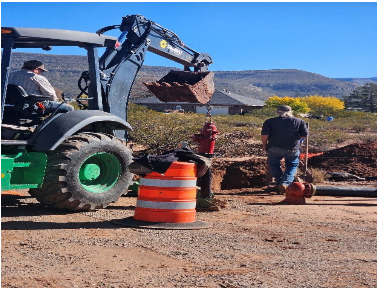
La Luz MDWC&MSWA Waterline and Hydrant Replacement
