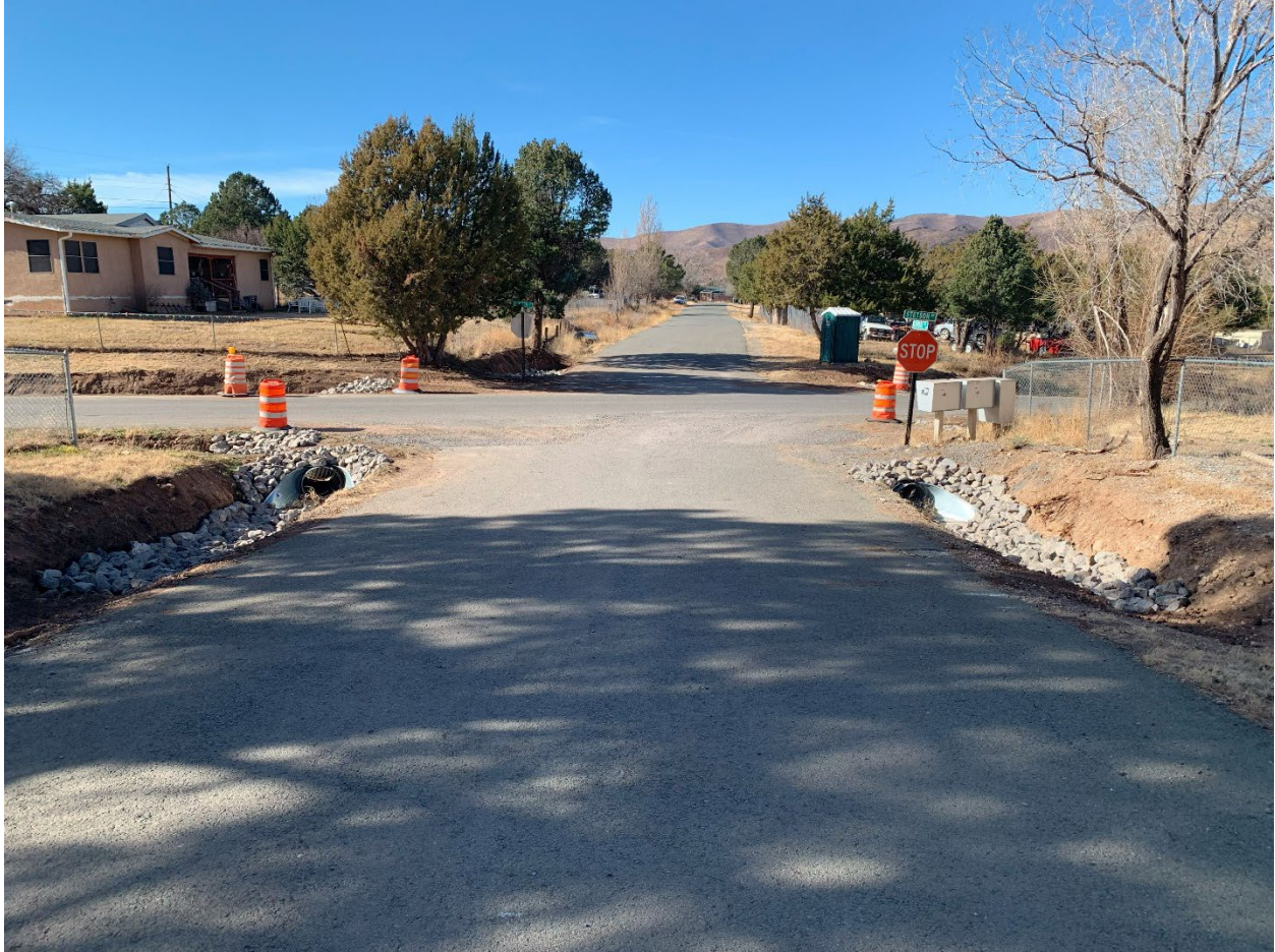
Lincoln County – Subsurface Stormwater Drainage Project
