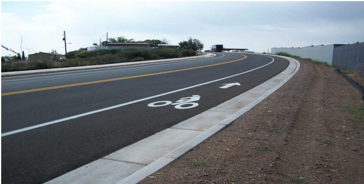
Town of Silver City – Ridge Road Street and Drainage Improvements
