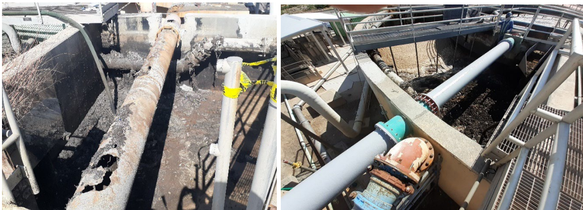
Camino Real Regional Utility Authority – Sunland Park Wastewater Treatment Plant Project
