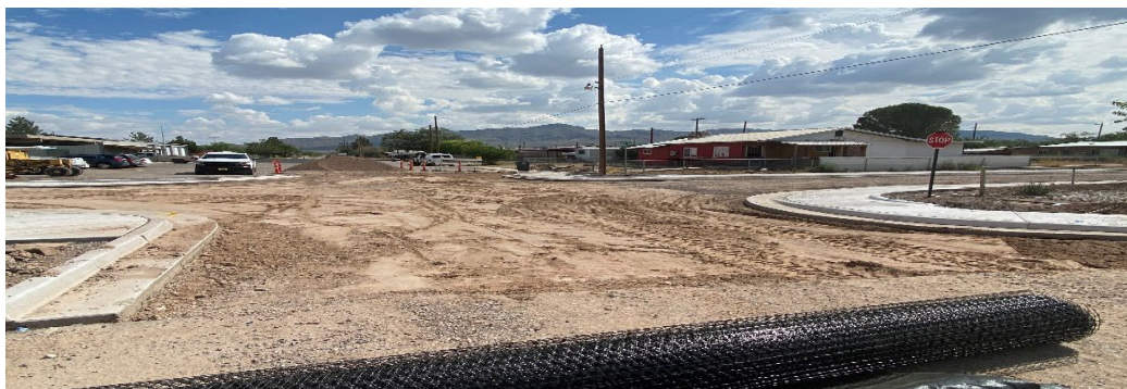
Village of Williamsburg – Mona and Doris Ave. Road and Drainage Project
